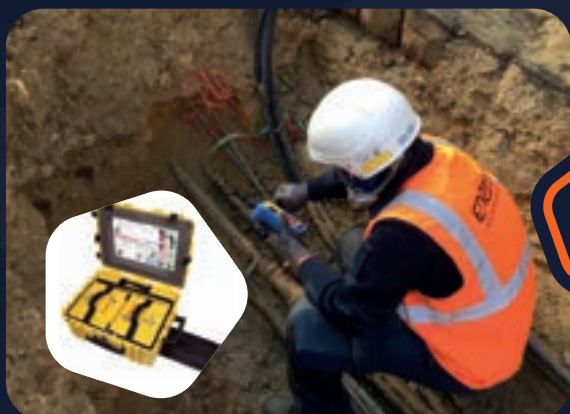
De-energized and dual grounded.
